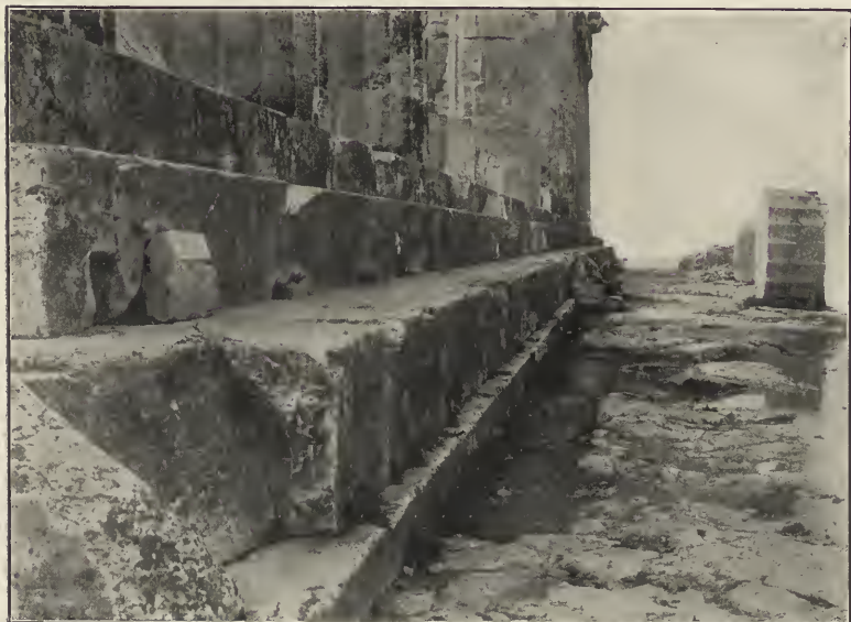
FIG. 49.—North Side of Parthenon, showing Curvature of Horizontal Lines.
